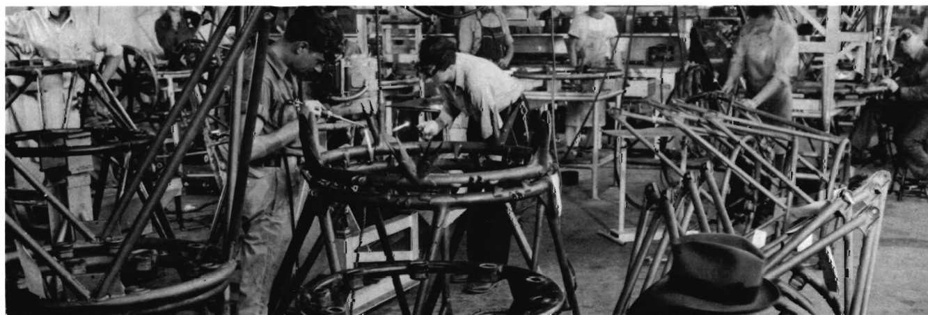
View in Douglas Engine Mount Welding Department
