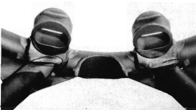
Figure No. 1A—Welding Cracks on Engine Mount Shown Up by Magnaflux Inspection.
